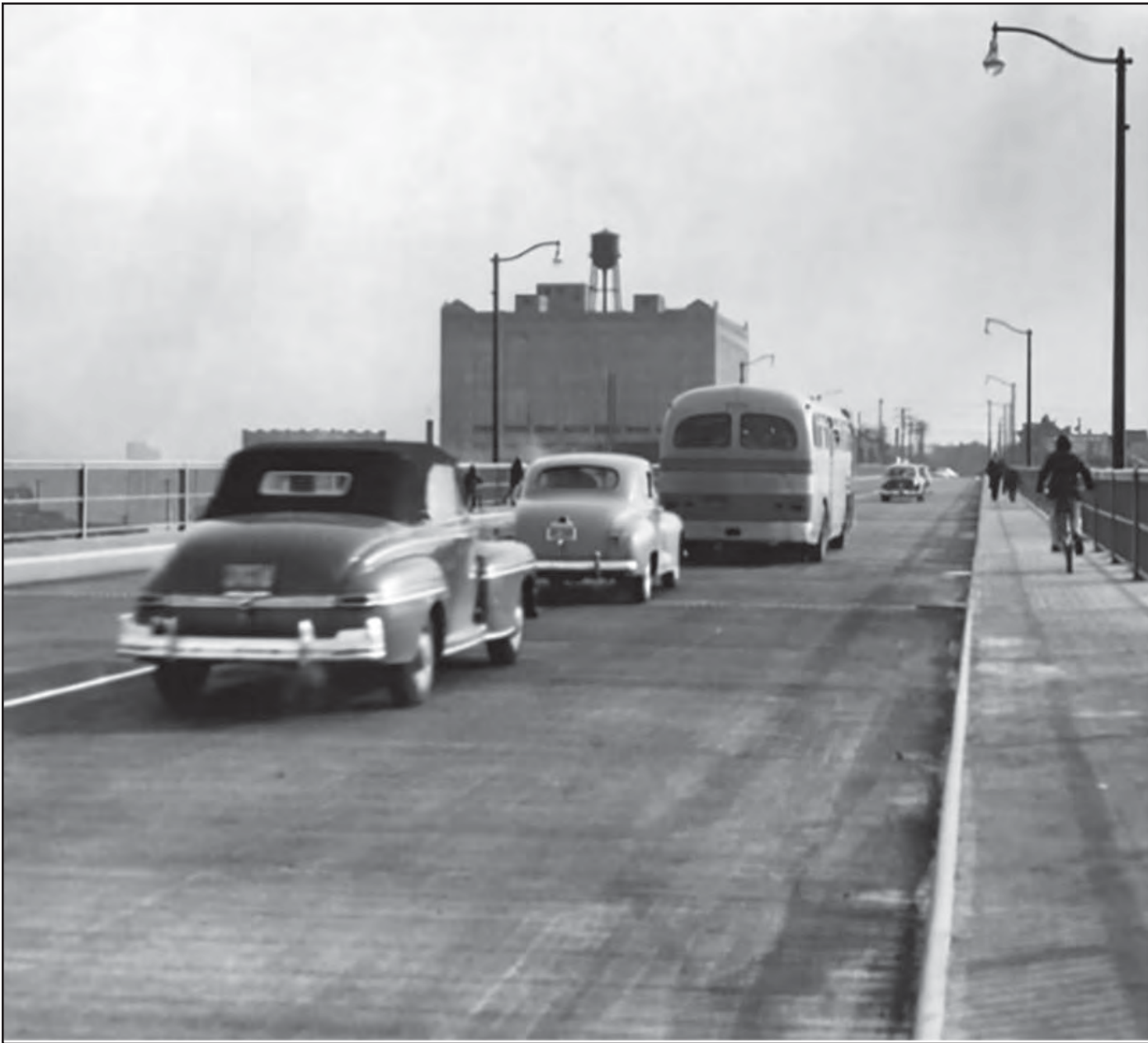
Old Abbey Ave. Bridge Looking East (photos courtesy of Ken Scigulinsky)
